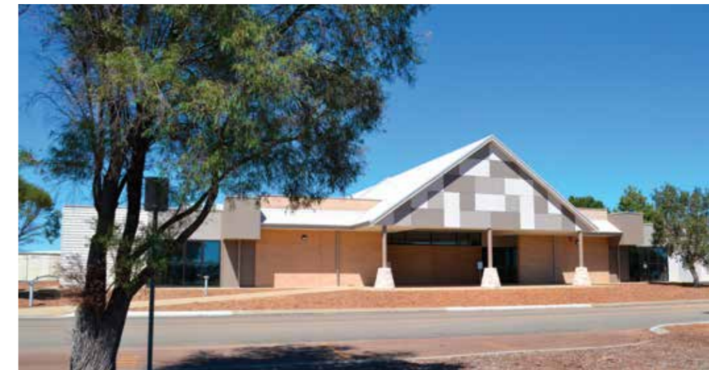
Busselton Airport Expansion Image of terminal building, photo courtesy of Busselton Airport.
